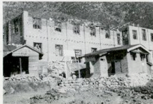
Building under Construction
