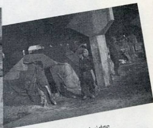
Under a bridge
