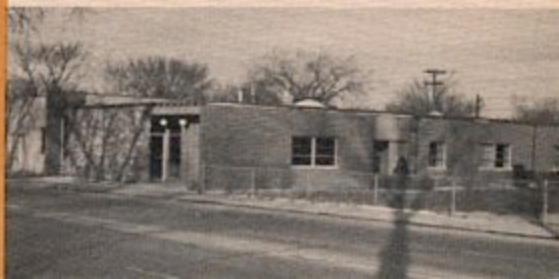
Headquarters Building located at 7774 Irving Park Road, Chicago.
