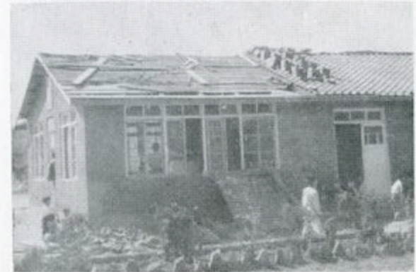
Building destroyed by typhoon being repaired Holy Lamp Orphanage.
