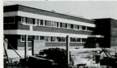
Construction progressed during Fall of 1966.
