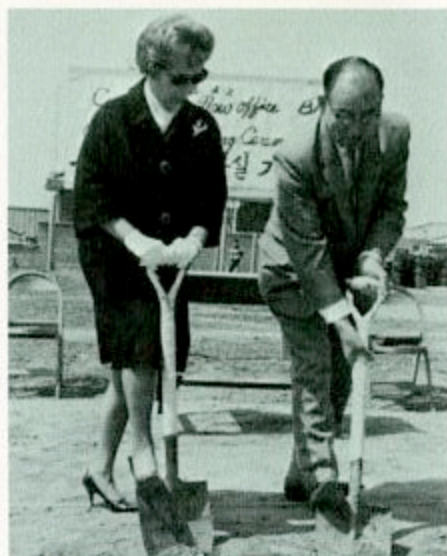
First shovel of ground removed, April, 1966.
