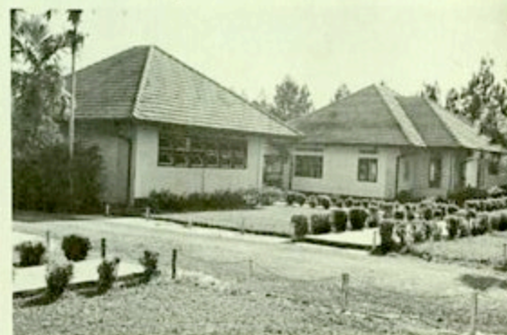
Classroom buildings at the Bible School
