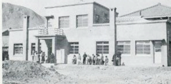
The Love Valley Orphanage was formerly using a Korean house and was extremely crowded. Now they have these completely new facilities. The cost was $5,600 plus $1,500 for garden land.
